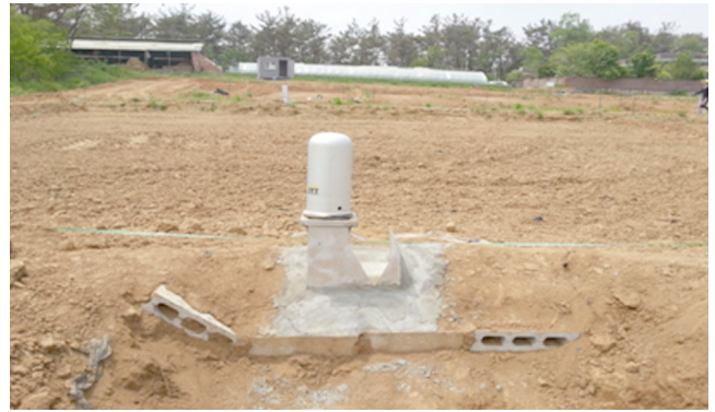
Fig. 3 Water level gauge
